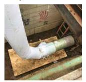
Aegion continues to advance the pipeline rehabilitation market by offering the latest innovations in cured-in-place pipe (CIPP) technology specifically engineered for drinking water applications. The InsituMain<sup>™</sup> System, our showcase CIPP innovation for pressure pipe renewal, is a composite material of polyester fiber, fiberglass, and a specially formulated epoxy resin system.
