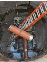
NO-DIG jacking pipe from Logan Clay Products is preferred for Pilot Tube Method of Guided Boring installations. Vitrified clay jacking pipe provides unsurpassed axial strength of 18,000 psi and greater. VCP-J eliminates the need for a casing pipe that remains in the ground. See a sample in booth #707.
