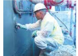
GeoCast™ Geopolymer Mortar is a microsilica geopolymer with fly-ash binder, pozzolan powder, polymer-modified and fib-r reinforced mixture with select admixtures for rehabilitation of horizontal concrete pipes, corrugated steel culverts, sewer manholes, and water treatment plant structures. The chemical resistant GeoCast™ withstands hydrogen sulfide corrosion and offers special additives for marine environments.
