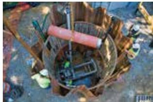
NO-DIG jacking pipe from Logan Clay Products is the preferred pipe for installations using the pilot tube method of guided boring. Vitrified clay jacking pipe provides unsurpassed axial strength of approximately 18,000 psi. See a sample (including the jointing system) in booth #620.
